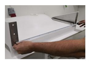
4. Measure where the operating sink should be located. The recommended height is 950 mm from the floor, note that it is 20 mm from the top hole and up to the top of the bracket and there should be 785 mm on the single sink between the brackets, from hole to hole.
