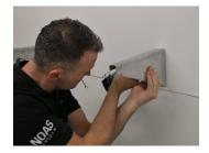
5. Insert the brackets into Solder and screw in all screws. Between the holes that are below each other on the console it is 65 mm. On the Double sink there are three brackets of which the middle is put in the middle (between the rounds see picture last page)
